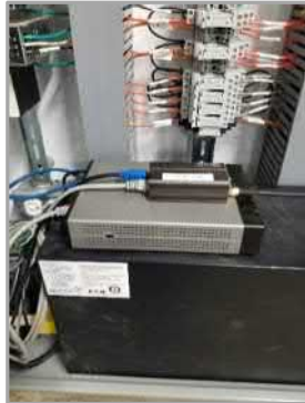
Cellular Modem and Router
