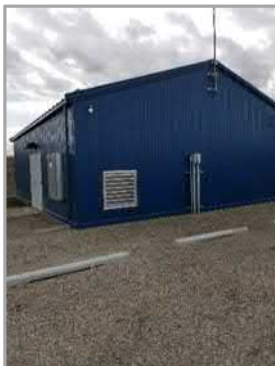
Radio Mast & Power Service
