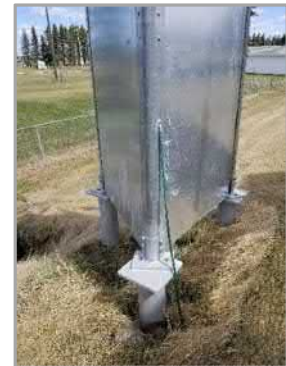
Radio Tower Grounding
