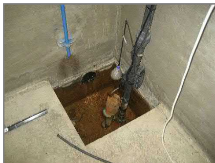
Image Table 2-15 HWY 21 Booster Station – Piping and Valves
