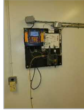
Cl2 Analyser and CO Detector
