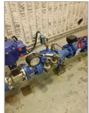
Valve and PRV Assembly
