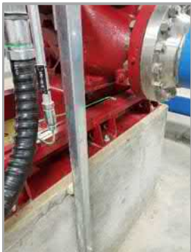
Pump Bonding
