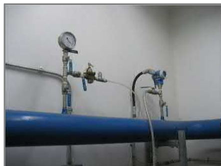
Remove Galvanized Fittings
