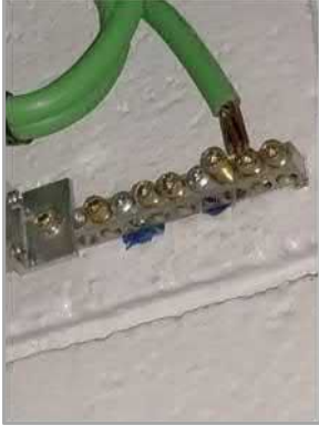
Ground Not Connected
