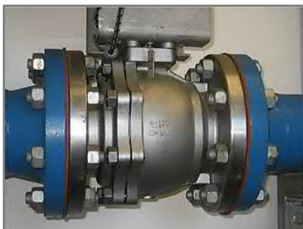
Flow Control Valve Reversed
