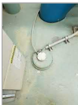
Level Element and CL2 drain
