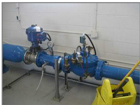
Piping, Valves Condition
