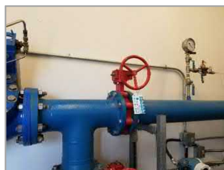
Bypass Isolation Valve
