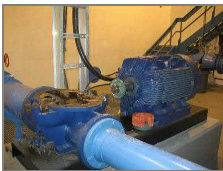
P-102 Dismantled for Service
