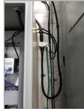
Radio Antenna Polyphaser
