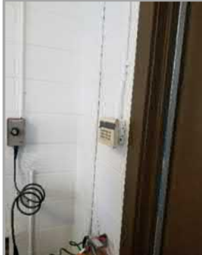
Heat Trace Controller & Keypad
