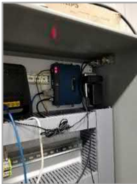
Cell Modem (left) and Radio
