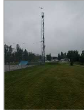
Antenna and Tower
