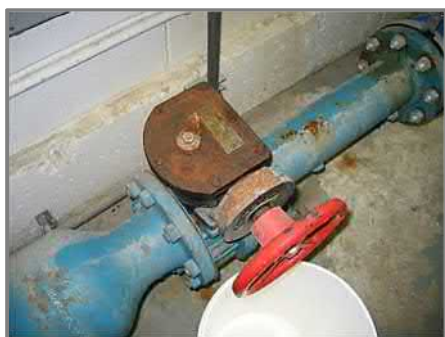
Significant Corrosion
