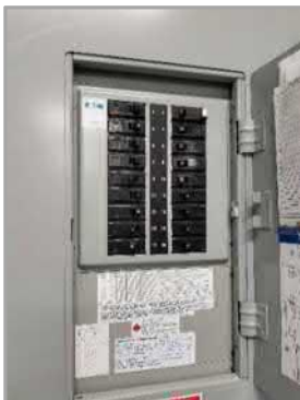
Distribution Panel; Sched is Blank
