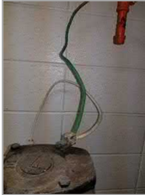
Ground Connection to Valve
