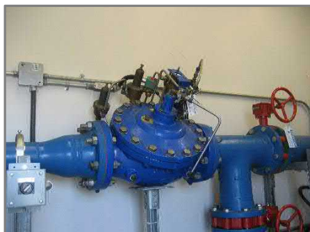
Pipe, Valves Condition
