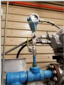
Pressure Transmitter
