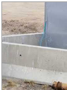
Radio Tower Grounding
