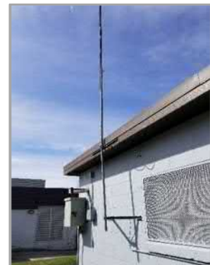
Cathodic Box & Antenna Mast
